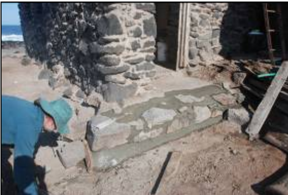
New step to support hut corner and organizing timber pile at back of hut
